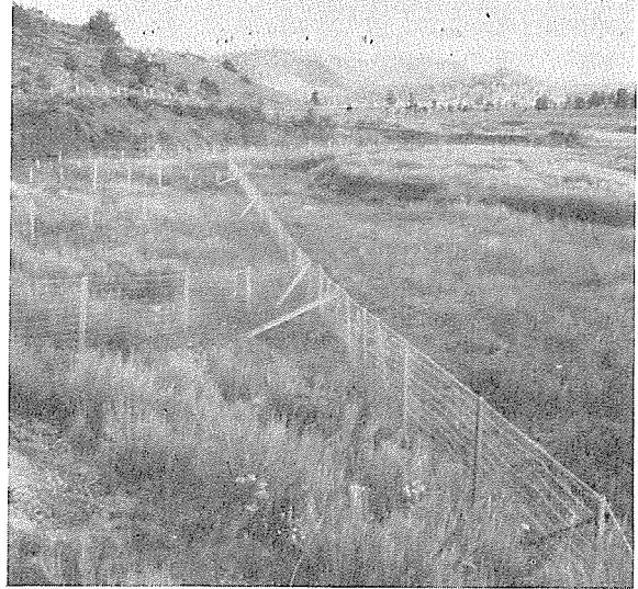
Figure 7. Working with the stream energy to stabilize bank cutting.
